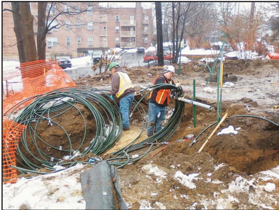
Photo 5: Oxygen Line Installation
