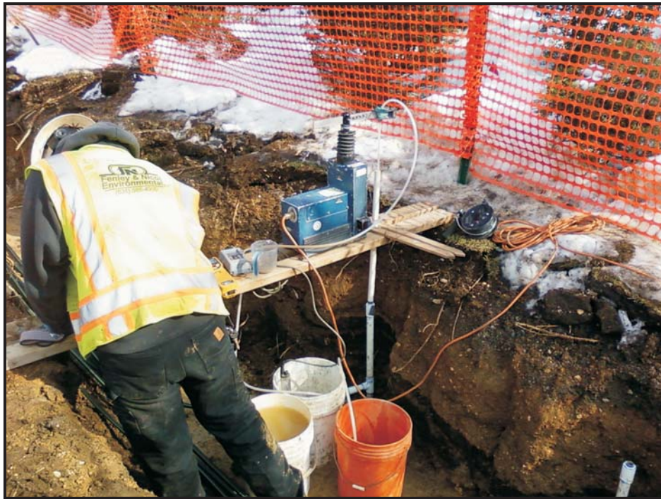
Photo 7: Oxygen Line Installation
