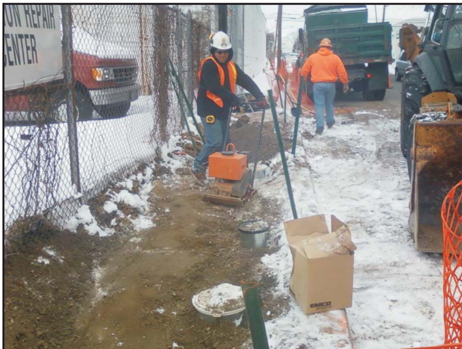
Photo 14: Compaction
