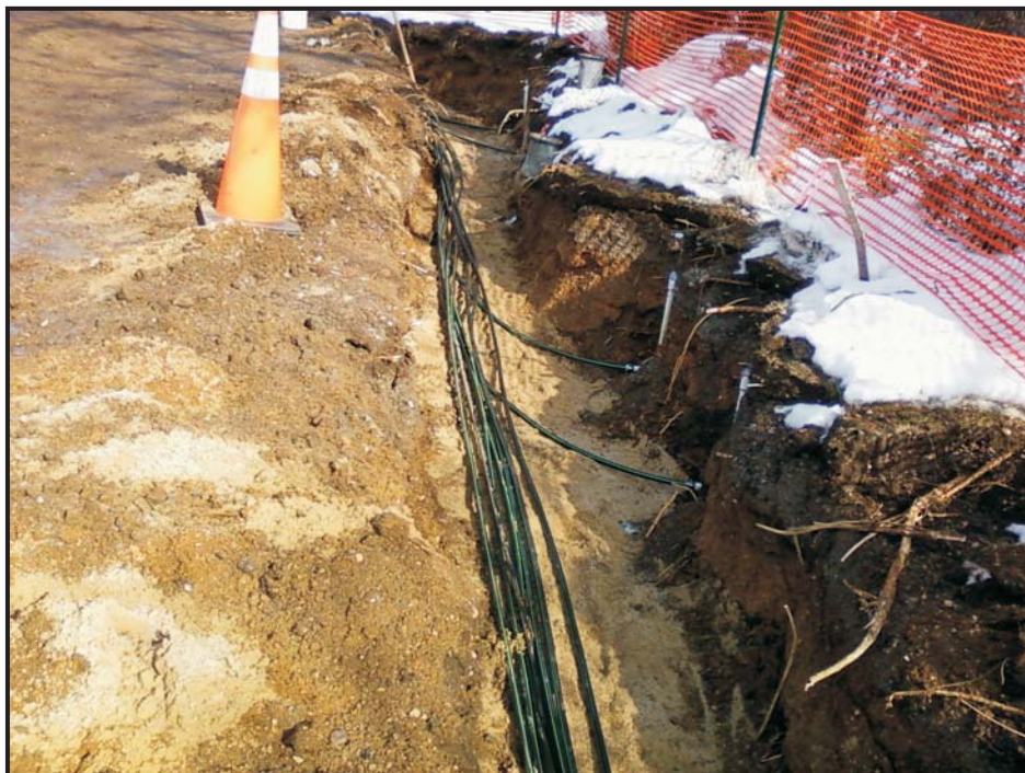
Photo 8: Oxygen Line Installation
