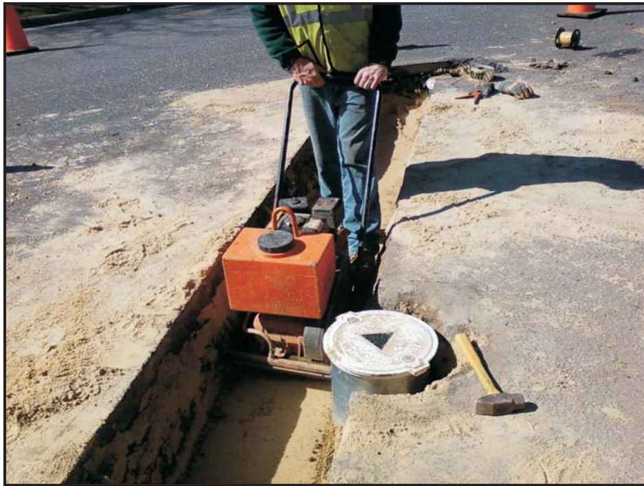
Photo 11: Compaction
