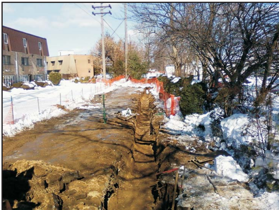
Photo 4: Trench Excavation
