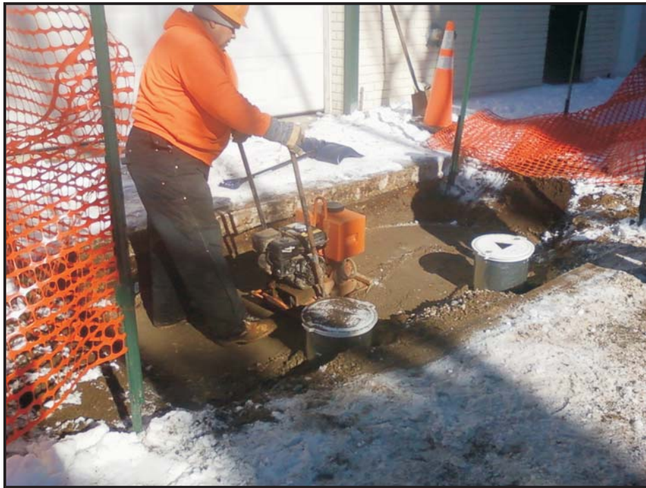
Photo 13: Compaction
