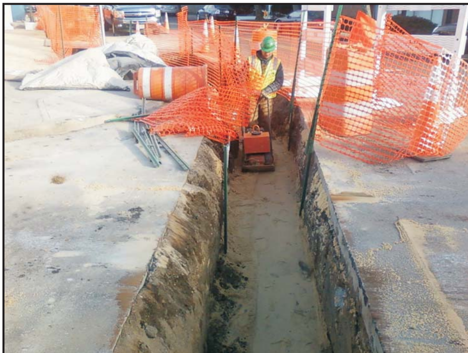
Photo 12: Compaction
