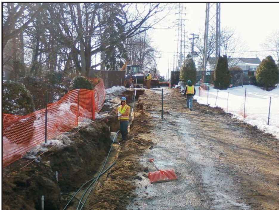
Photo 6: Oxygen Line Installation
