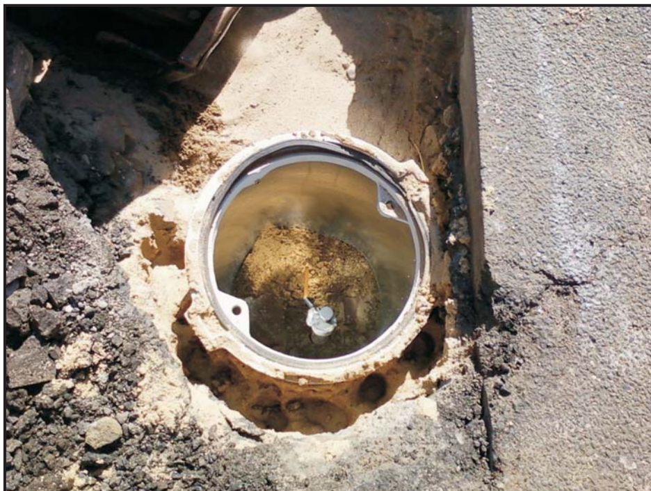
Photo 10: Oxygen Line Installation
