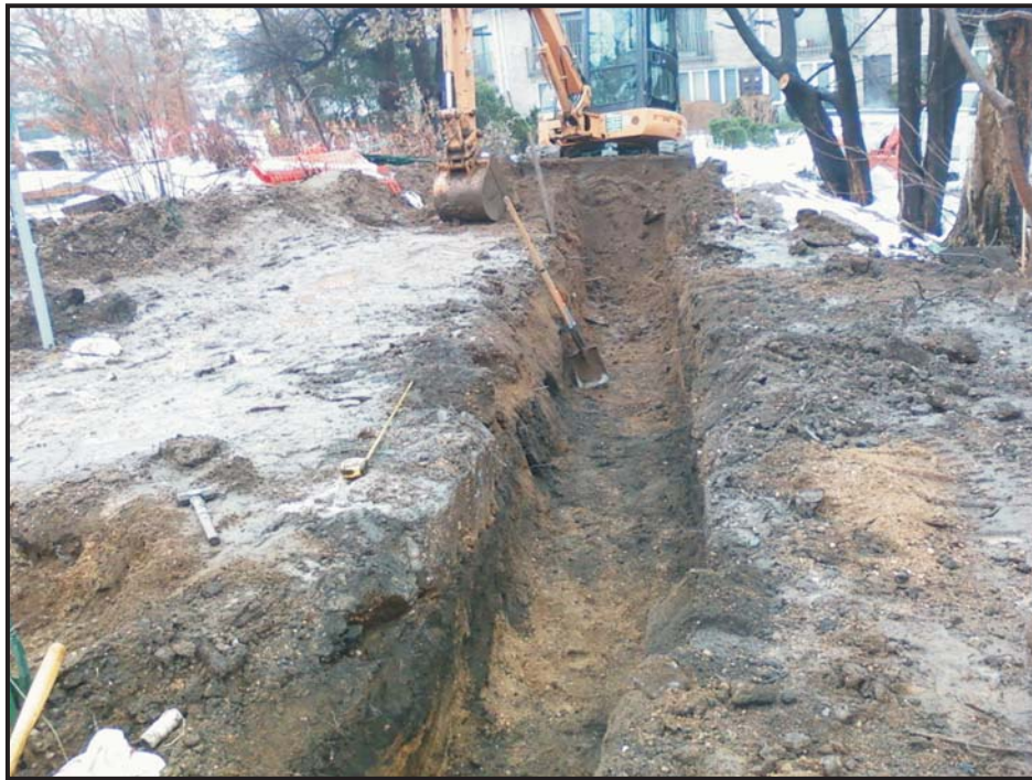
Photo 3: Trench Excavation
